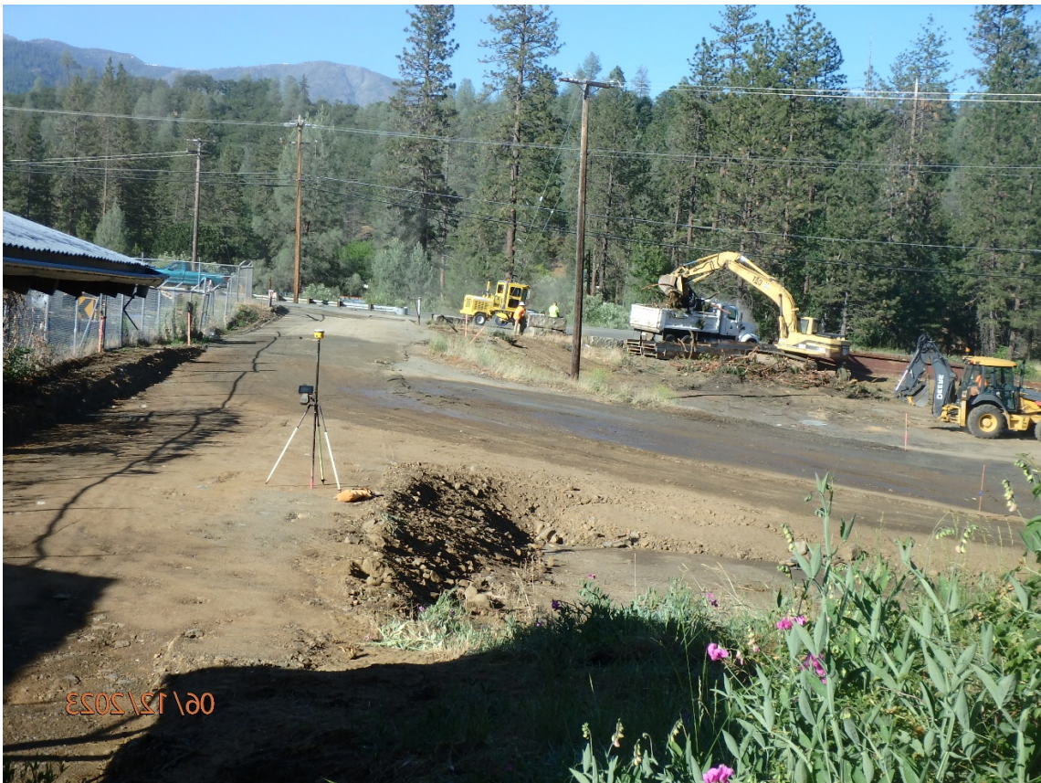
Transit Parking Lot cleanup by County crews prior to construction
