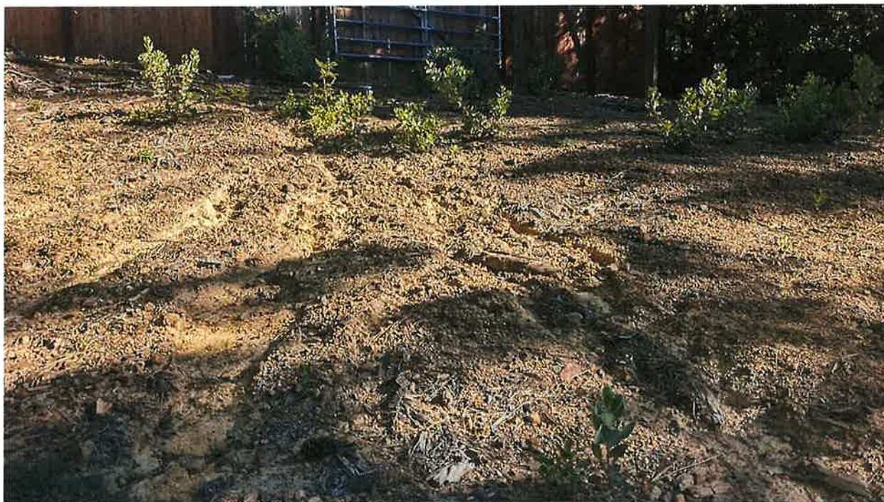
Figure 12: July 2023 photograph of runoff from NatureFarm property causing erosion on adjacent property still visible in late-summer.
