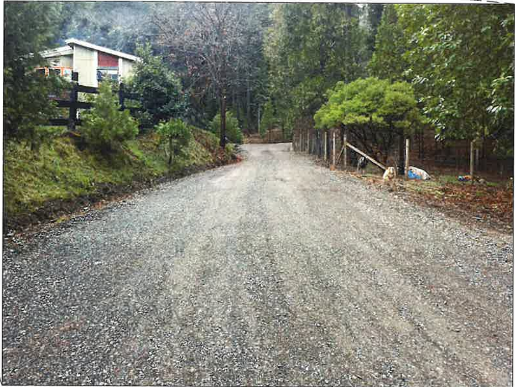
EXISTING ROAD LOOKING SOUTHWEST NTS
