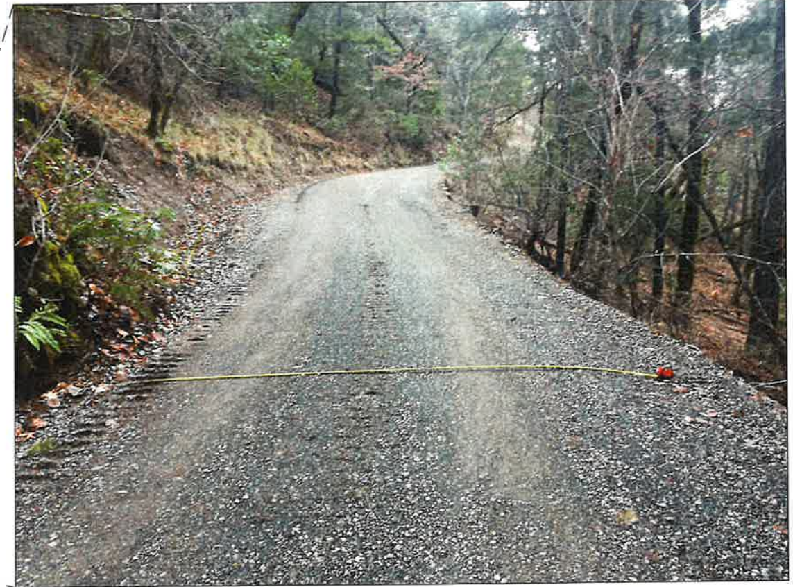
EXISTING ROAD LOOKING NORTHWEST NTS
