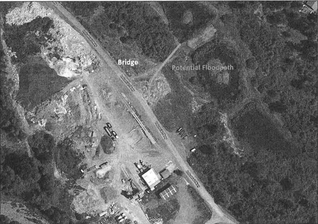
Compromised Levee allowing excess water to enter wetlands
