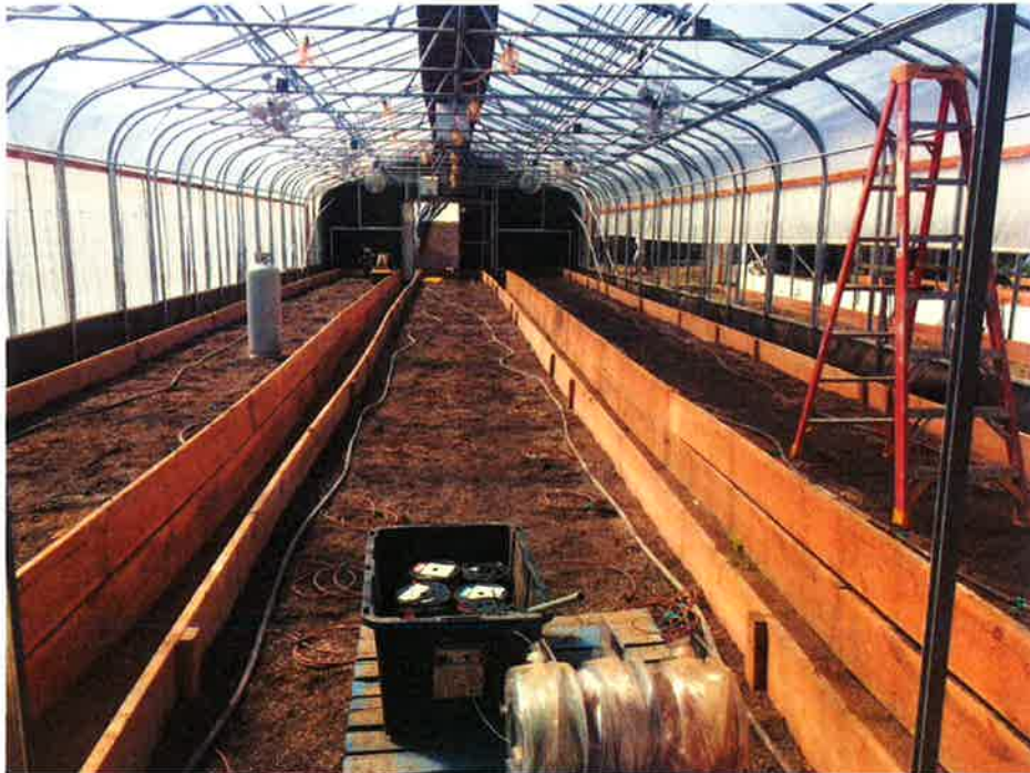
Picture 3: Interior picture of one of the two (2) newly constructed Greenhouses within the 350 ft. residential buffer. Both Greenhouses were permitted and built to code.
