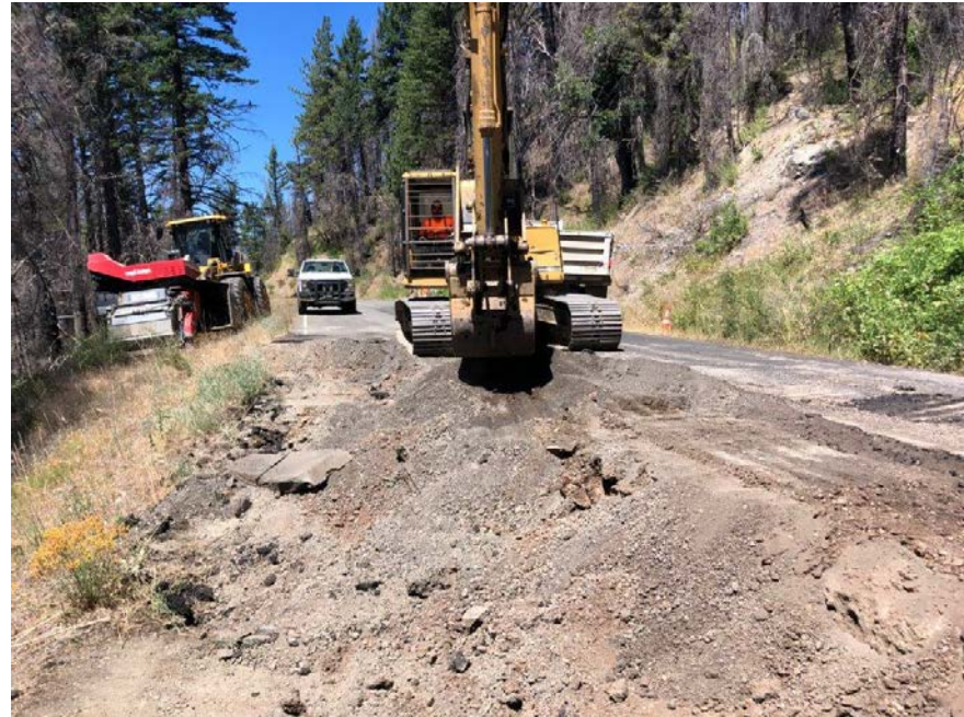
Ruth Zenia MP 18.6 Excavating Slip-out
