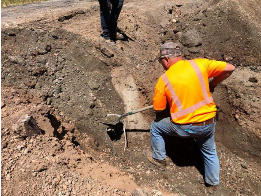
Ruth Zenia MP 18.6 Pipe repairs
