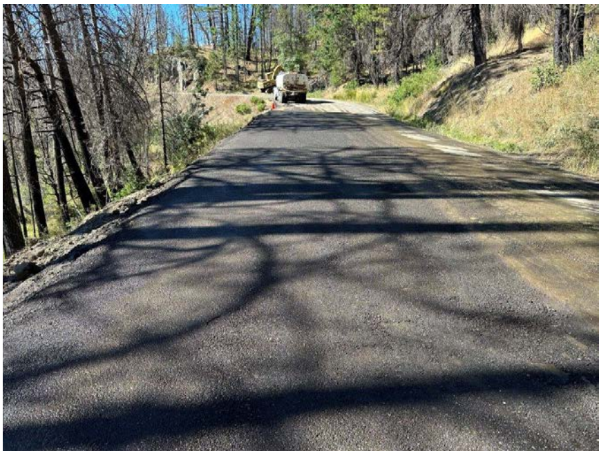
Ruth Zenia MP 18.6 Temporary Repair (grindings)
