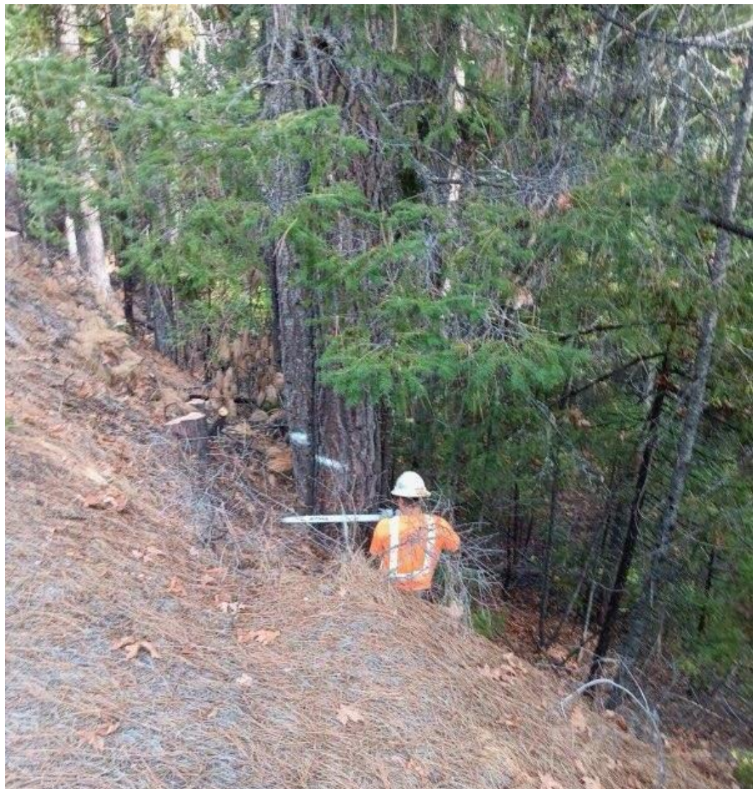
Hazardous tree removal by DOT crews on Trinity Dam Blvd.
