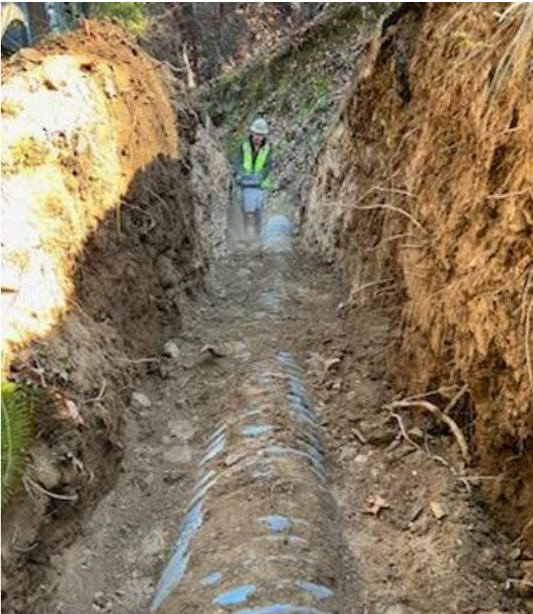
Replacing burned culverts by DOT crews on Campbell Ridge Rd. and New Snowblower on the Multihog
