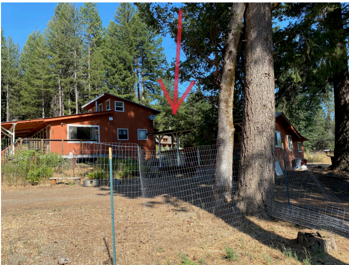
<-- Residence Located on APN 016-200-008
