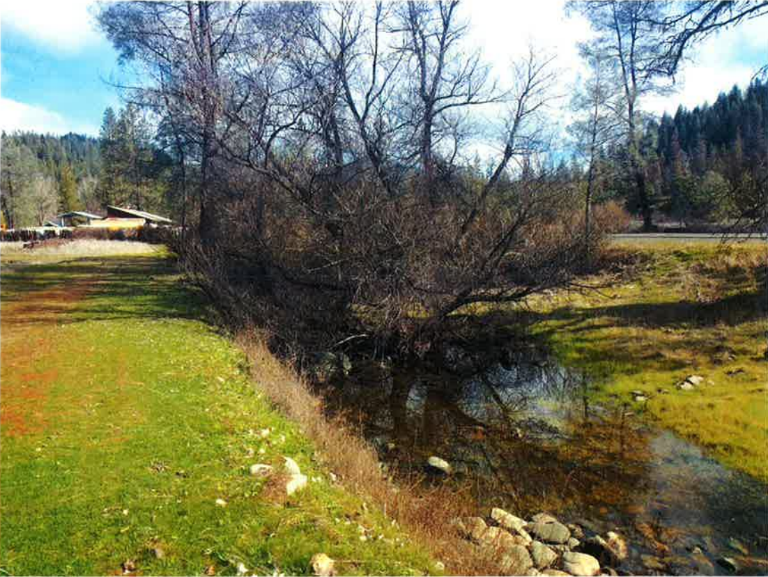
Figure 4a – Ditch between subject parcels and Highway 3 – looking north towards vehicle yard
