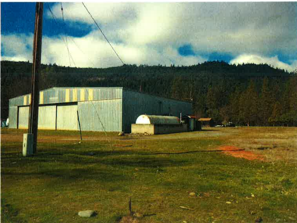
Figure 4d – Existing building on APN 015-490-10, with tank on right. Looking west
