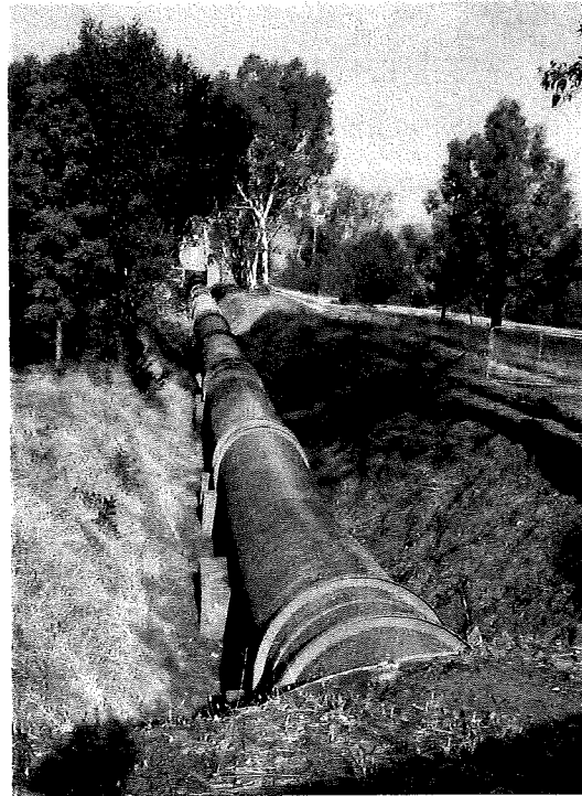
South Feather Water and Power Agency's Kelly Ridge Powerhouse penstock. Photo courtesy of the Butte County Department of Development Services.
