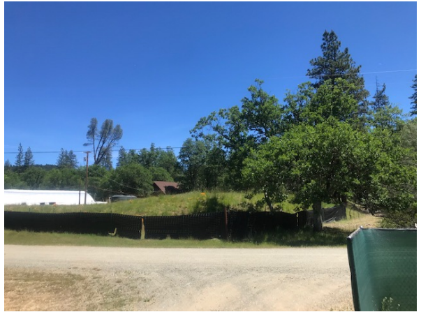
View of Residence Located on APN 014-290-02-00
