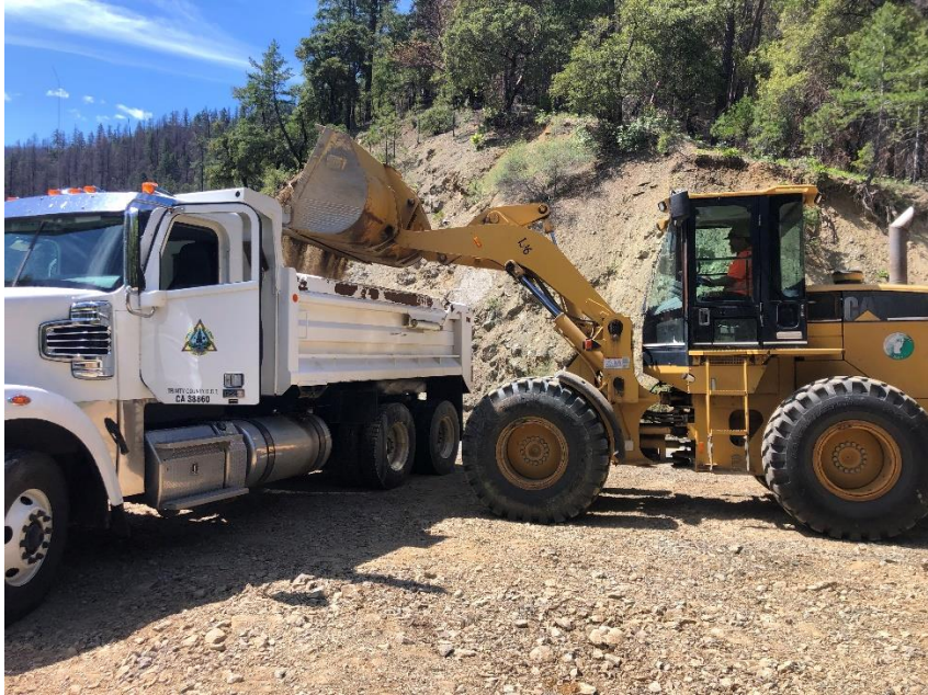
Loading and hauling off slide material in multiple locations, along Hyampom Road
