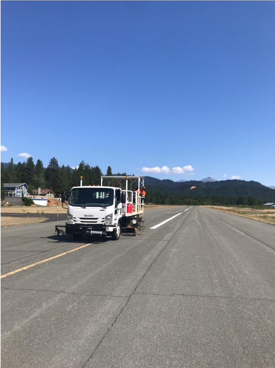
County crews are paving a centerline stripe at the Trinity Center Airport
