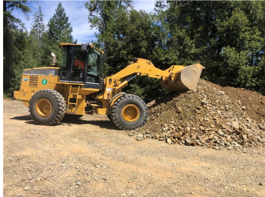
Loading and hauling off slide material in multiple locations, along Hyampom Road
