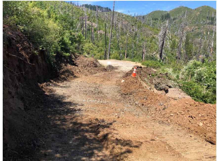
Opening up Lower Southfork Road at PM 10.5 and starting the cut for a new road
