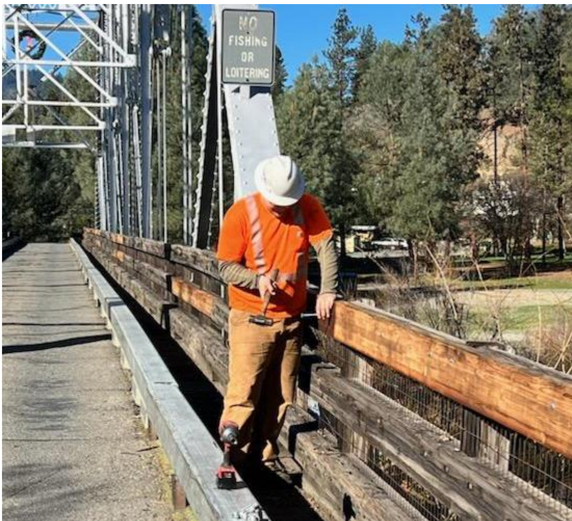
County Crews Repairing Damage Boards on the Lewiston Historic Bridge
