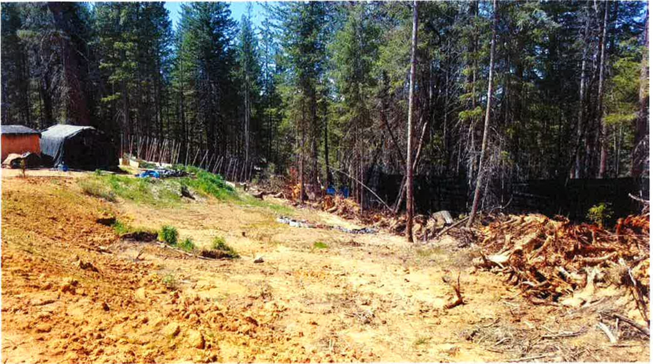
Picture 5: facing north-west towards clearing debris
