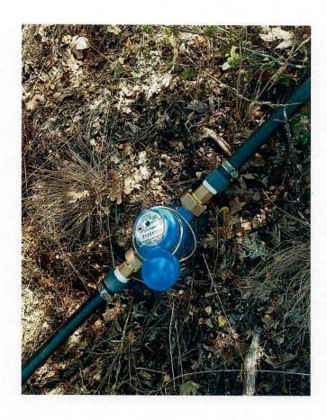
Water meter installed on main water line from well house to holding tank.
