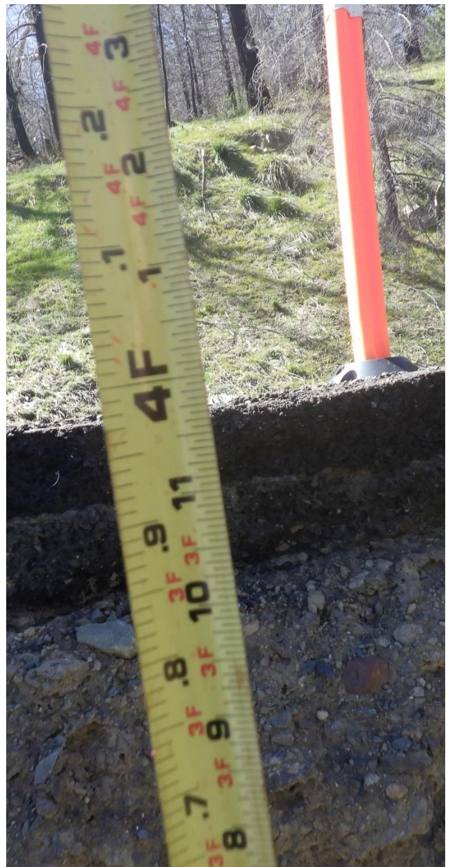
Typical depth of failures at above site
