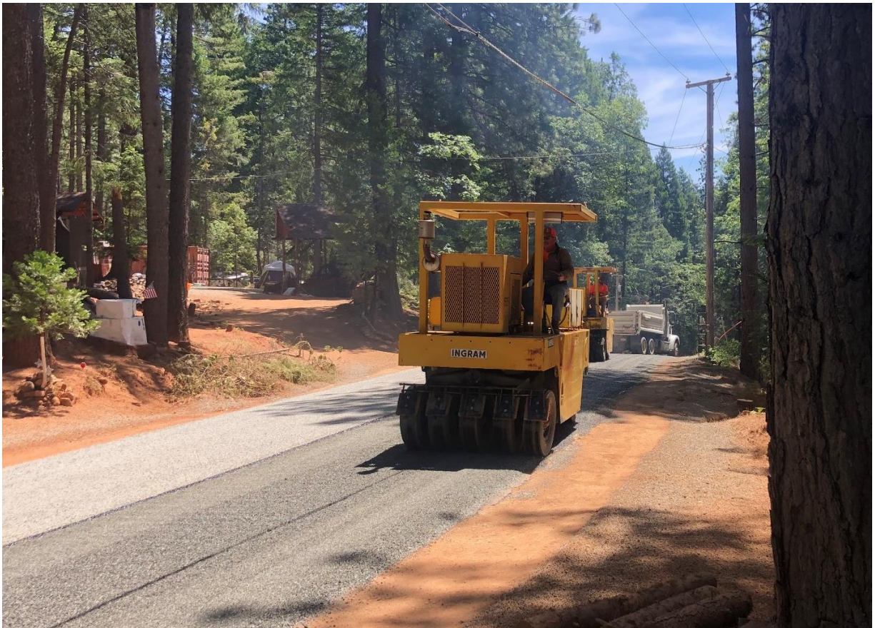
Chip Seal operations by County crews on Lake Forest
