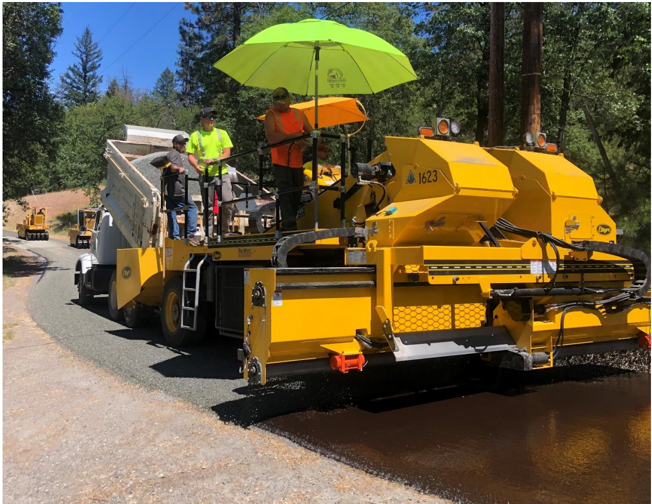
Chip Seal operations by County crews on Mountain View Drive
