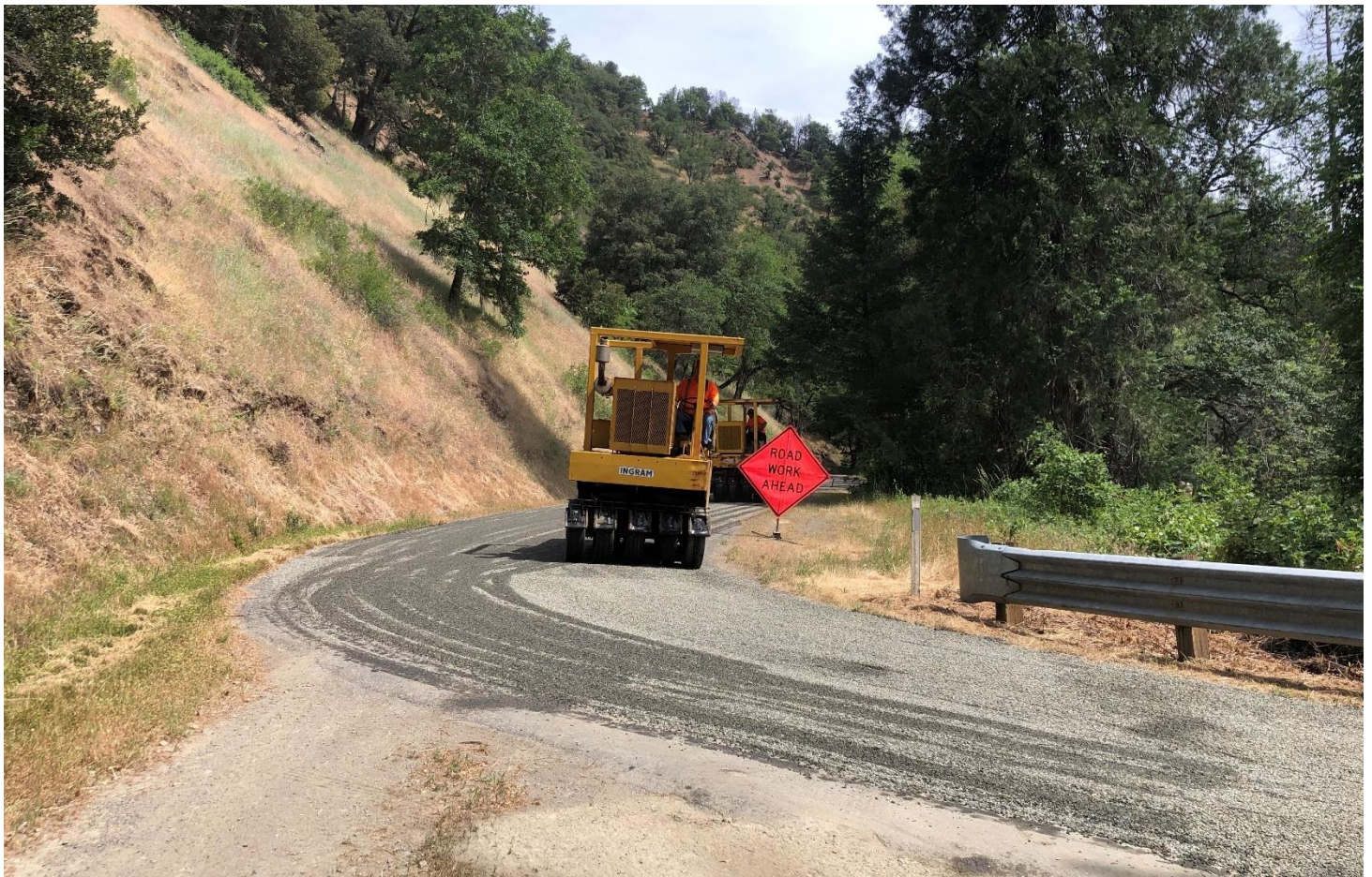
Chip Seal on B-Bar-K Road
