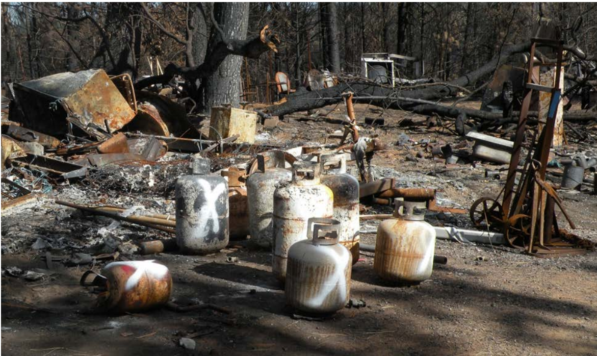
Miscellaneous Tanks De-headed and Marked with a White "X."
