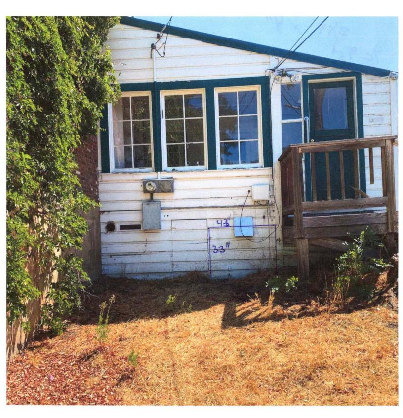
Under the proposed location for the condenser unit of the HVAC, I was going to pour a 2" X 4" slab for it.
